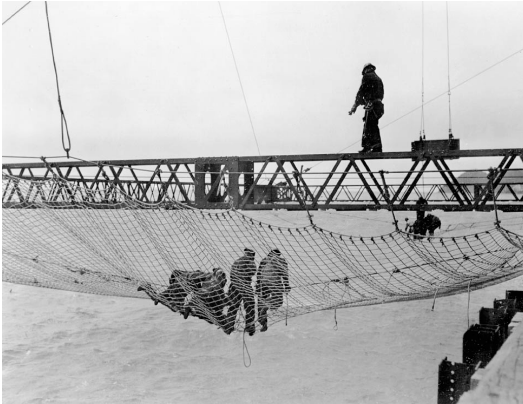
Fig. 4. Strauss's safety net Golden Gate Bridge, Highway & Transportation District. Golden Gate Bridge Construction Safety Net .
