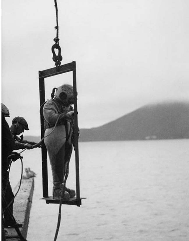
Fig. 2. Diver holding an air hose ready to be lowered into water at the Golden Gate Huggins, Ted. Diver, Golden Gate Bridge construction . 1933-34.
