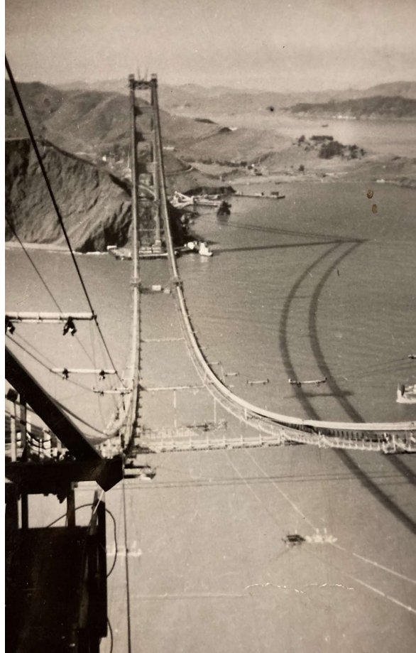
Fig. 3. The Golden Gate Bridge with only suspension cables and towers Dondero, George. Photo of the Golden Gate Bridge during construction. 1935.
